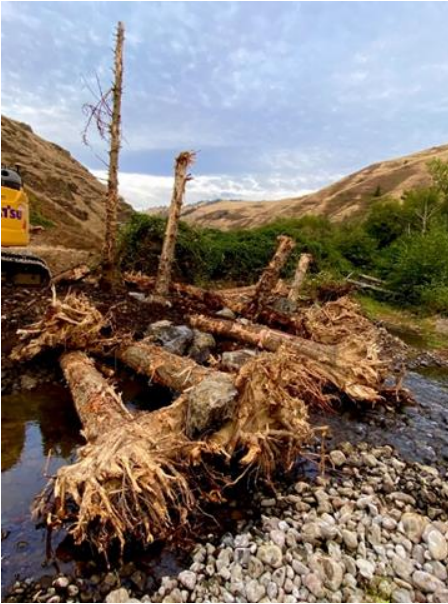
Figure 29. ELJ configurations were strategically constructed to reduce buoyancy and remain intact during high flow events.
