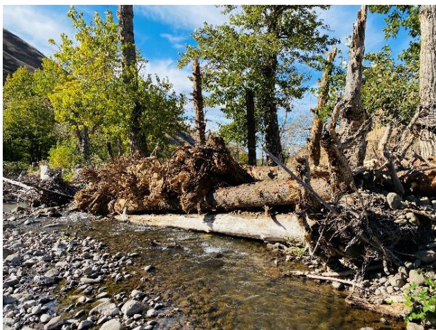
Figure 27. ELJ Bank Structure near RM 4.1 provided quality fish habitat uplift.
