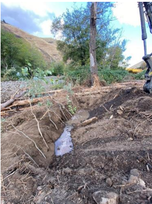
Figure 38. Trenching technique for planting willow and cottonwood cuttings in contact with water table.
