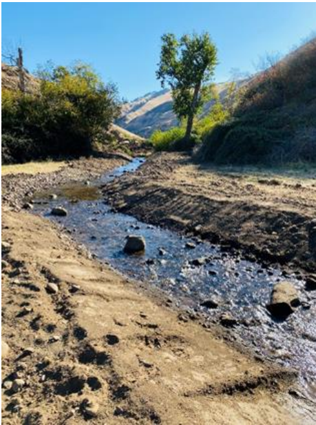
Figure 37. North Fork Walla Walla River RM 5.2 after implementation.
