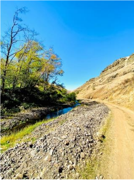
Figure 35. NFWWR RM 5.1 side channel following construction.
