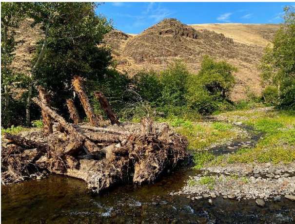
Figure 42. Roughness elements added to barren gravel bars to promote retention of fine sediments, point bar development, and riparian recovery.
